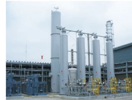
PSA装置 設計圧力:1.6MPaG 処理量:1,000m 3 /h PSA system Design Pressure: 1.6MPaG Processing Capacity: 1,000m 3 /h
