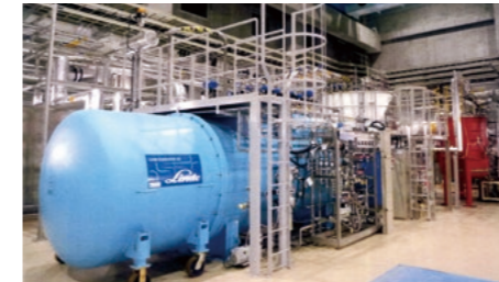
ヘリウム冷凍機 (TCF200S) 冷凍能力: 1,200W at 4.5K 2,400W below 80K 1.1g/s at 4.5K
